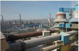
Material will be feed into kiln tail through chute in gas chamber. As kiln shell is inclined and it rotates slightly, material will move along round shell and will also move along shaft direction from kiln tail to kiln head. Material will be processed through pre-heat, decompose, calcined and will be feed into cooler. Fuel will be
