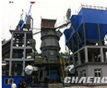
300,000t/a GGBS Production Line of Tangshan Hongyan Building Material.
