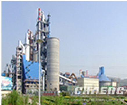
1.5 Million t/a GGBS Plant of Baosteel Group Corporation
