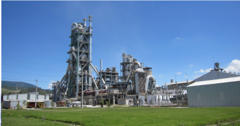
3500t/d cement line in Albania
